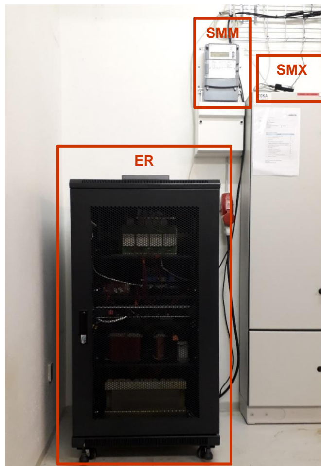
Figure 1. Three-phase ER and USM deployed in the residential test site (Skive, DK).
